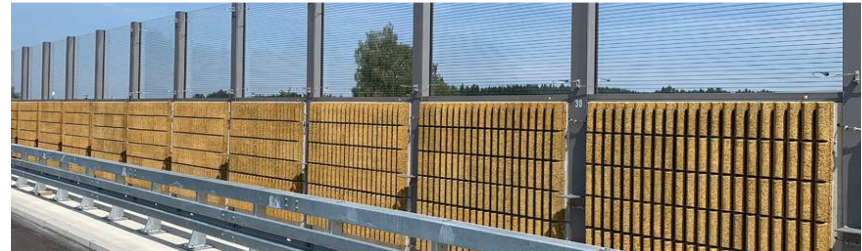
D-PPP A94, Mühldorf, Forstinning-Marktl, KOHLHAUER SCORSA® FRAME made of GS CC combined with concrete elements
