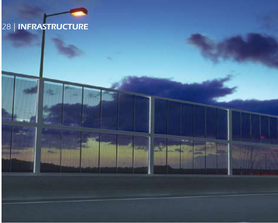
This barrier features solar technology to help reduce the infrastructure carbon footprint
